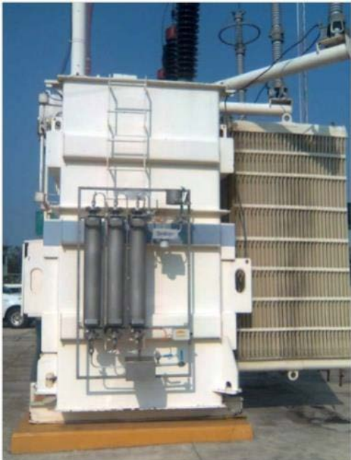
Figure 2: DryKeep® installed directly on transformer
