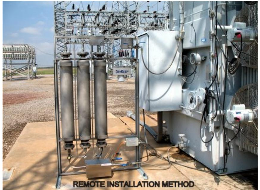
Figure 3: Installation adjacent to transformer on customer-fabricated free-standing frame
