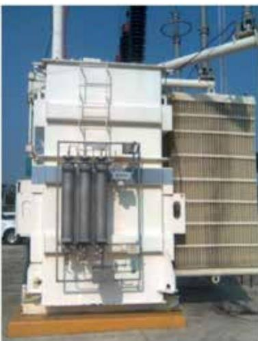
Condition based maintenance with DryKeep® can extend the operational life of a power transformer by years.
