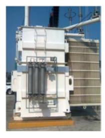
Condition based maintenance with DryKeep® can extend the operational life of a power transformer by years.
