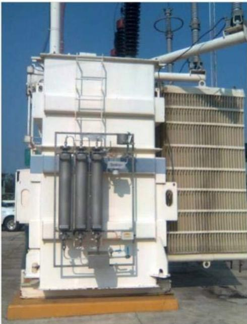
Figure 2: DryKeep® installed directly on transformer
