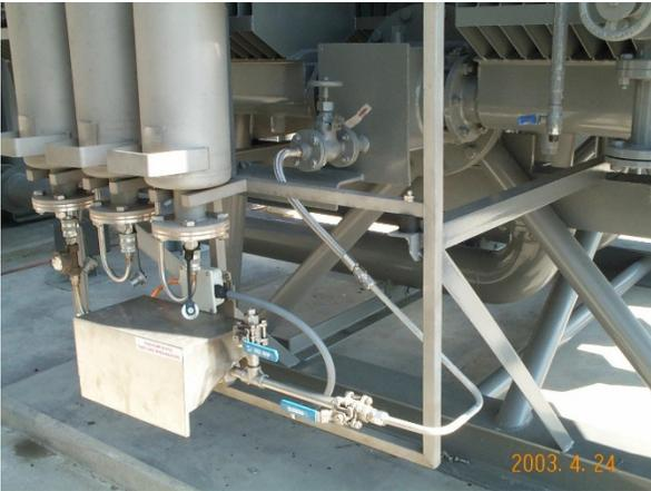
Figure 4: Connection from transformer to DryKeep® inlet valve.
