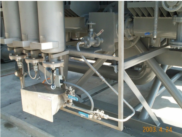
Figure 4: Connection from transformer to DryKeep® inlet valve.
