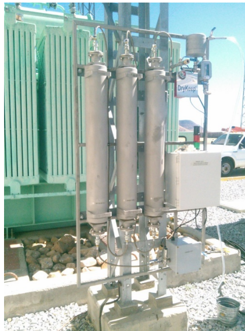
Figure 3: Installation adjacent to transformer on customer-fabricated free-standing frame
