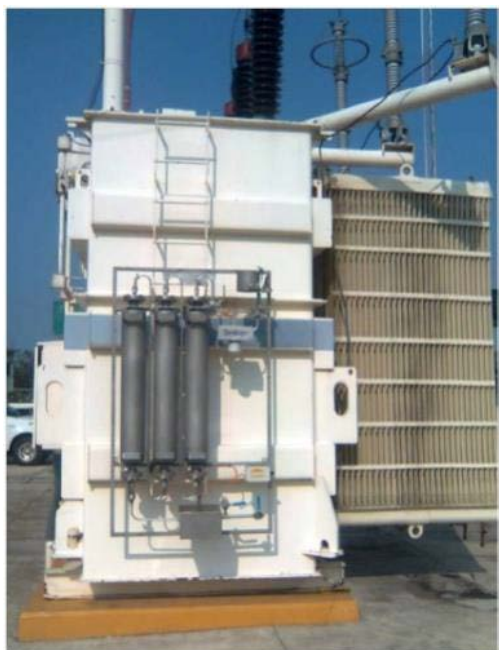
Figure 2: DryKeep® installed directly on transformer
