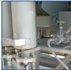
**Installation Kit** Two (2) stainless steel transformer valve flange adapters to customer's provided dimensions. Two (2) 0.44" O.D. static dissipative core tube, 304 stainless steel braided, PTFE hoses to SAE 100R14B standard with all necessary unions, bushings, and hardware for hose connections to connect DryKeep® inlet and outlet valves to the transformer.
